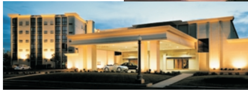
Design build lighting renovations— Holiday Inn. Sacramento, CA
